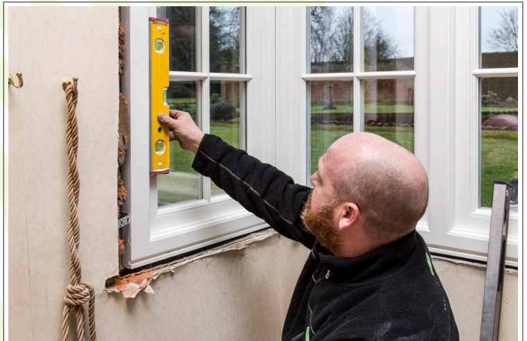
Windows and doors should be fitted plumb and square.
