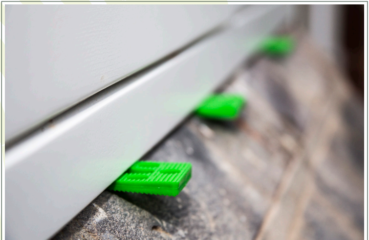
Packer or wedges should be used to level.
