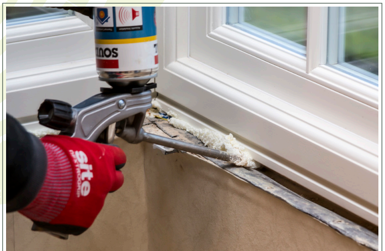
Small amounts of expanding foam to seal the perimeter.
